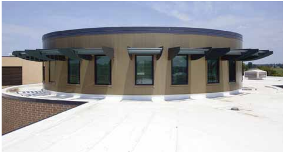
The simple action of using light-colored roofing materials reduces the absorption of solar radiation and the energy costs to counteract associated heating.
